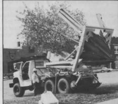
Vermeer Tree Spades. Patented tree-moving/tree-packaging machines that automatically dig, ball, transport and replant shrubs and trees up to 25 ft. in height. Tractor-mounted, trailer-mounted, or truck-mounted units—plus complete multi-purpose landscaping machines that handle a tremendous assortment of dirthandling functions in addition to transplanting trees.
