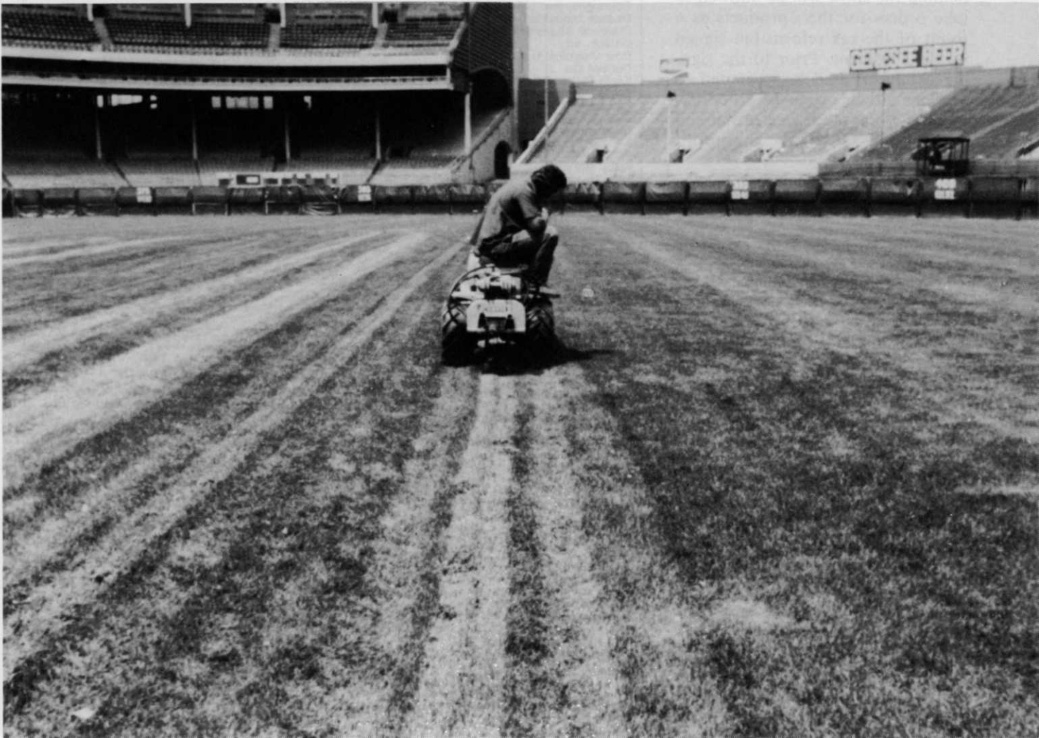
Installation in progress at Cleveland Stadium.
