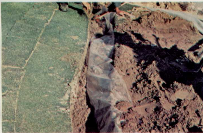
Top left, sod is removed. Top right, barrier, eight inches below surface is exposed. Lower left, plastic attached to original barrier is brought to surface. Lower right, sand is replaced and tamped for replacement of sod.
