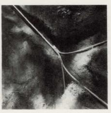
For lightning protection a special conductor cable is attached to the highest parts of the tree (left) and runs along major branches down the tree trunk. The ground system (right) consists of an extension of the main trunk cable to a point beyond the main root system and is attached to a rod driven to the required depth.
