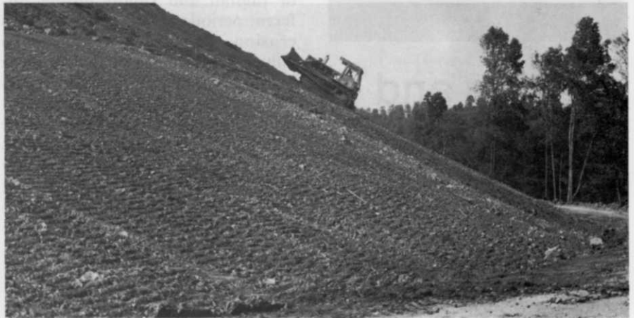
Grading for new vegetation — The Princess Susan Coal Corp., Charleston, W.Va.
