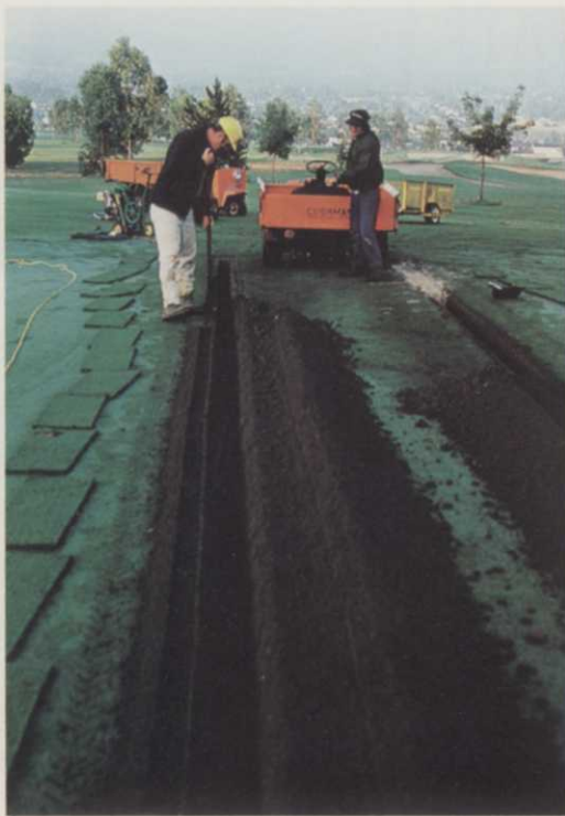
Ed Watson, golf course supervisor for the city of Walnut Creek, prepares one of the trench drains for a green (left), and after work has been completed (right).
