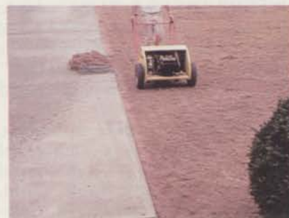
Plugging and debris removal.
