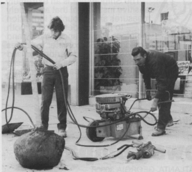
Two crew members prepare to chisel a hole through the sidewalk. The portable hydraulic unit is wheeled into position.
