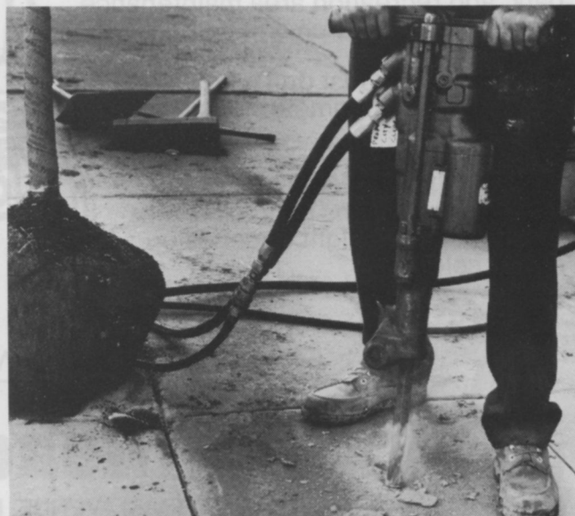
After the sidewalk has been scored and cut, the jackhammer is used to break-up the concrete.
