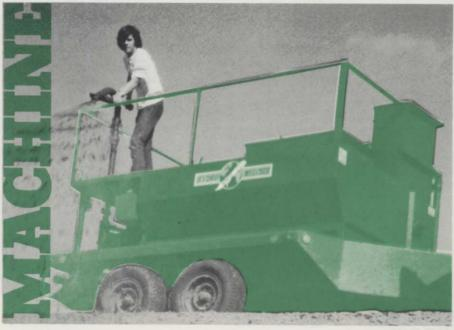
This is the machine that revolutionized the turf industry . . . the machine that seeds or sprigs, fertilizes, waters, sprays, and mulches in one easy operation . . . the BOWIE HYDRO-MULCHER.
