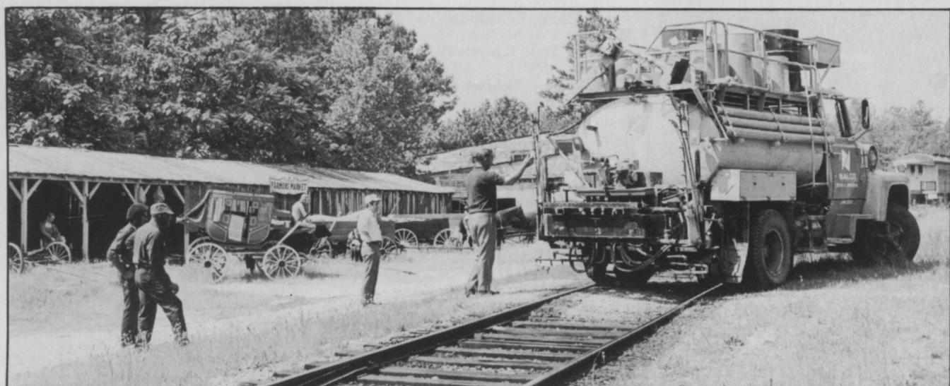
The Hi-Rail truck sets up to spray the residual herbicide and 2,4-D treatment. This versatile on-off track vehicle is faster and more efficient than the hand sprayers the railroad had been using. Background displays the "1880's motif" seen along the track.
