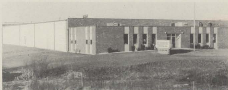
This new Hesston Lawn Equipment Division facility more than triples the division's production capacity and office space.
