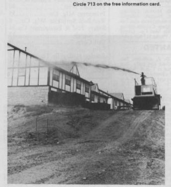
**HYDRO MULCH FIBERS:** Designed by Conwed to improve the hydraulic mulching process in areas of severe wind or water erosion. A soil stabilizer has been premixed with Hydro Mulch fibers; a uniform, weedfree fiber that helps foster good germination by retaining water and protecting seed from temperature extremes.
