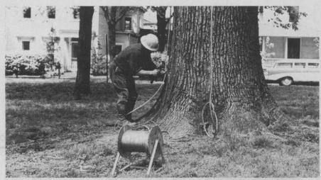
According to Code recommendations, two down-conductors are needed for large trees having trunks more than three feet in diameter. Cables lead from air terminals at top and on main branches to at least two grounds, located outside main root system.
