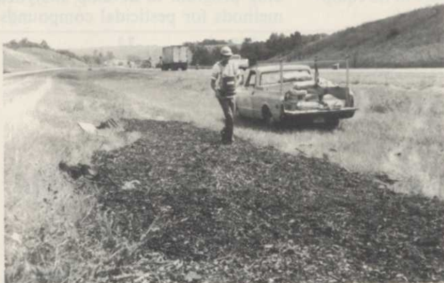
After chips are spread, fertilizer is broadcast over the top and the area is seeded.
