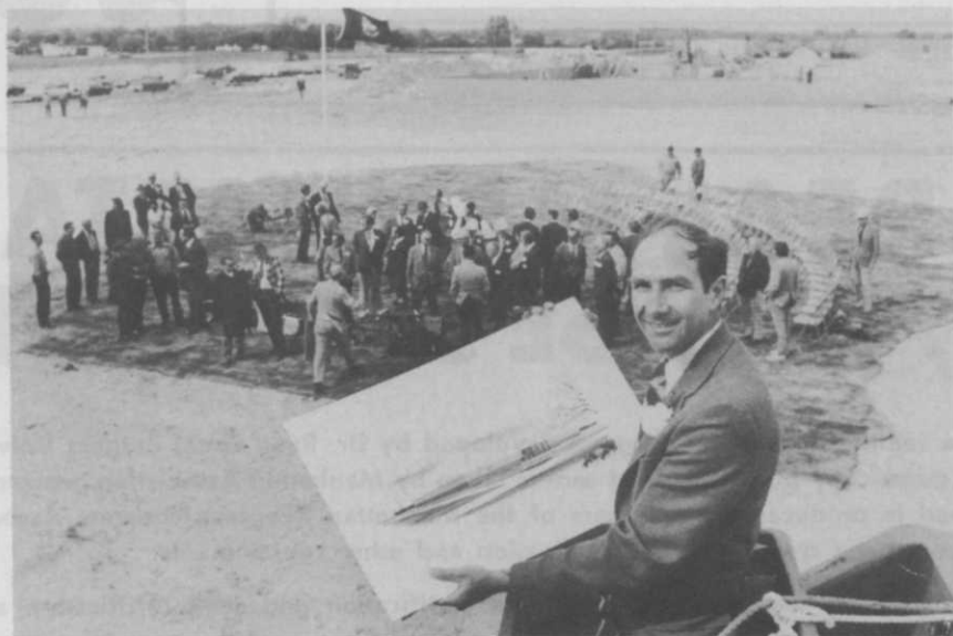
David T. McLaughlin, president of The Toro Company, holds a rendering of Toro's new assembly plant being built in Tomah, Wis.
