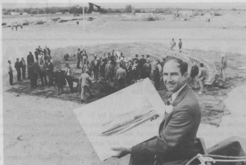
David T. McLaughlin, president of The Toro Company, holds a rendering of Toro's new assembly plant being built in Tomah, Wis.
