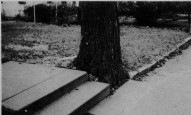
Improper location of street-side trees and short sighted planning can result in conditions like this.
