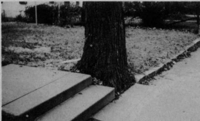
Improper location of street-side trees and short sighted planning can result in conditions like this.
