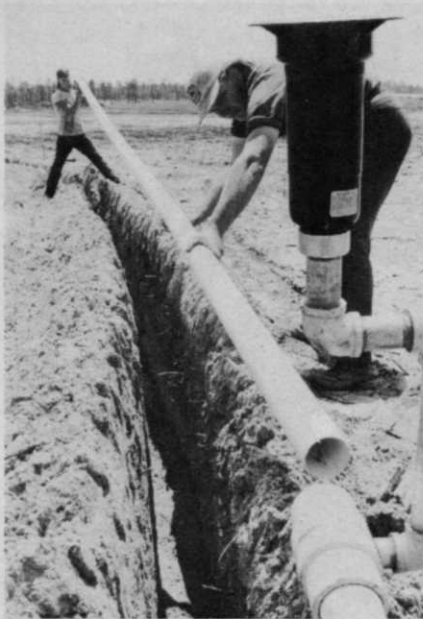
Two men join a 40 foot section of PVC pipe with another. It is linked to a sprinkler head on the edge of a green.
