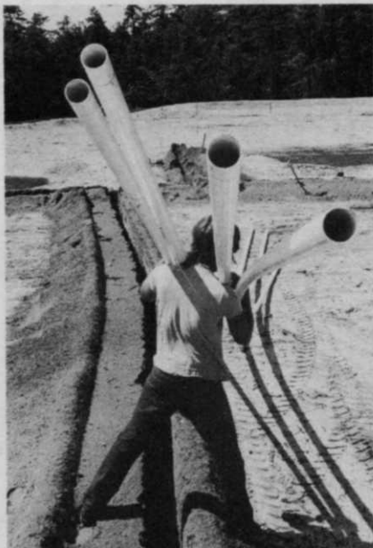
This pipe is light weight. One man can handle 40 foot sections with ease. No special handling equipment is needed.
