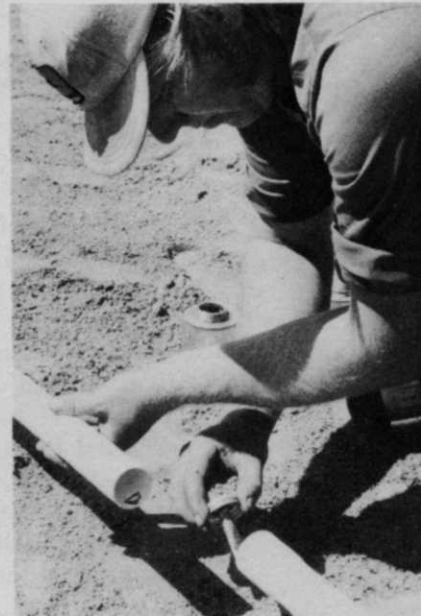
Solvent welds are completed in minutes. Interior of bell and end of one section is coated. Exterior of the spigot end is coated. Joining is done manually.
