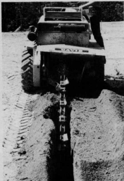
A trenching machine was the only piece of special equipment required to lay the irrigation system's pipe network.
