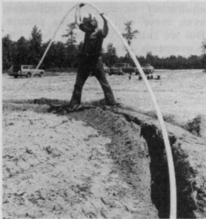
The flexibility of PPC means the pipe could easily bend around greens on King's Grant Golf Course.
