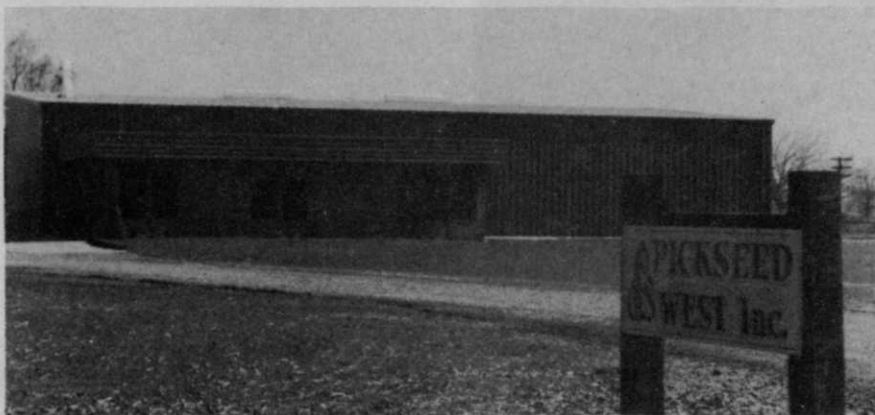
Pickseed West, Inc., plans to double this storage facility at Tangent, Ore.
