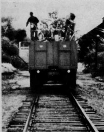
Visko-Rhap clears right of way along railroad tracks.
