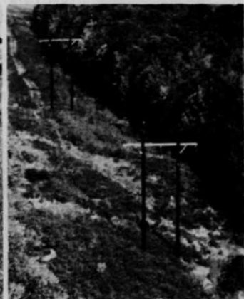
Power lines cleared by Visko-Rhap of unwanted foliage.
