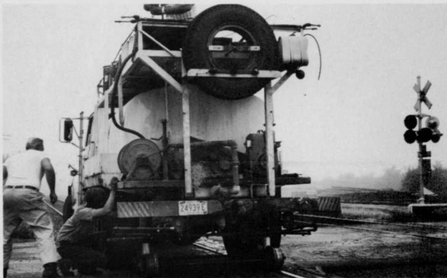
The on-off the track vehicle applies about 25 to 30 gallons per acre. In addition to being more economical than spray trains, they are more efficient and result in fewer claim damages.
