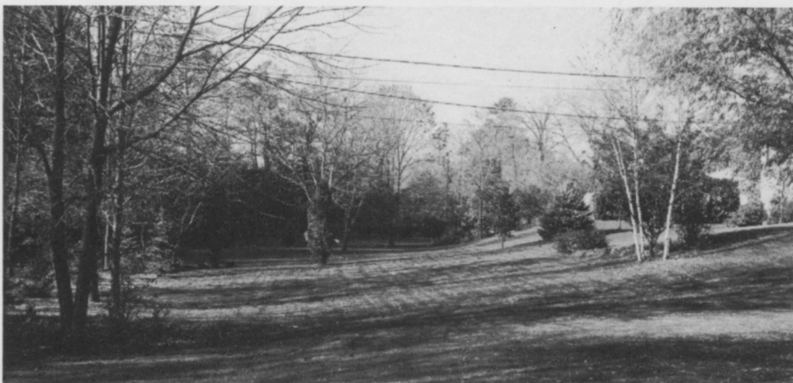
After construction and restoration, the area looked like this.
