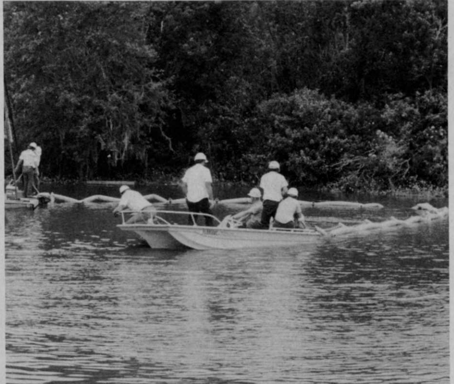
Work crews install a barrier by floating it into place and then tying it down to concrete blocks. Barrier is easy to maneuver.
