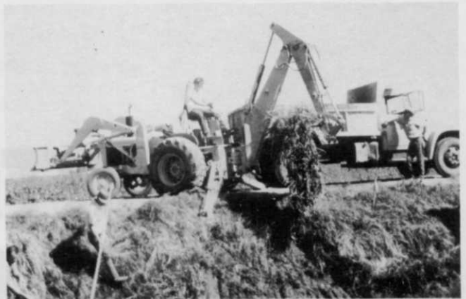
Work crews from the Lower Tule Irrigation District remove alligatorweed with a backhoe. Mats of the weed become so thick that water cannot flow along the ditches.
