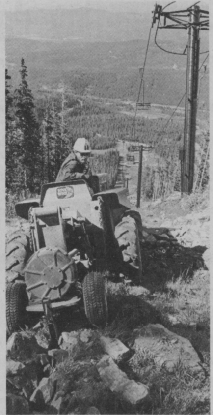
Operator breaks up rocks in first pass.
