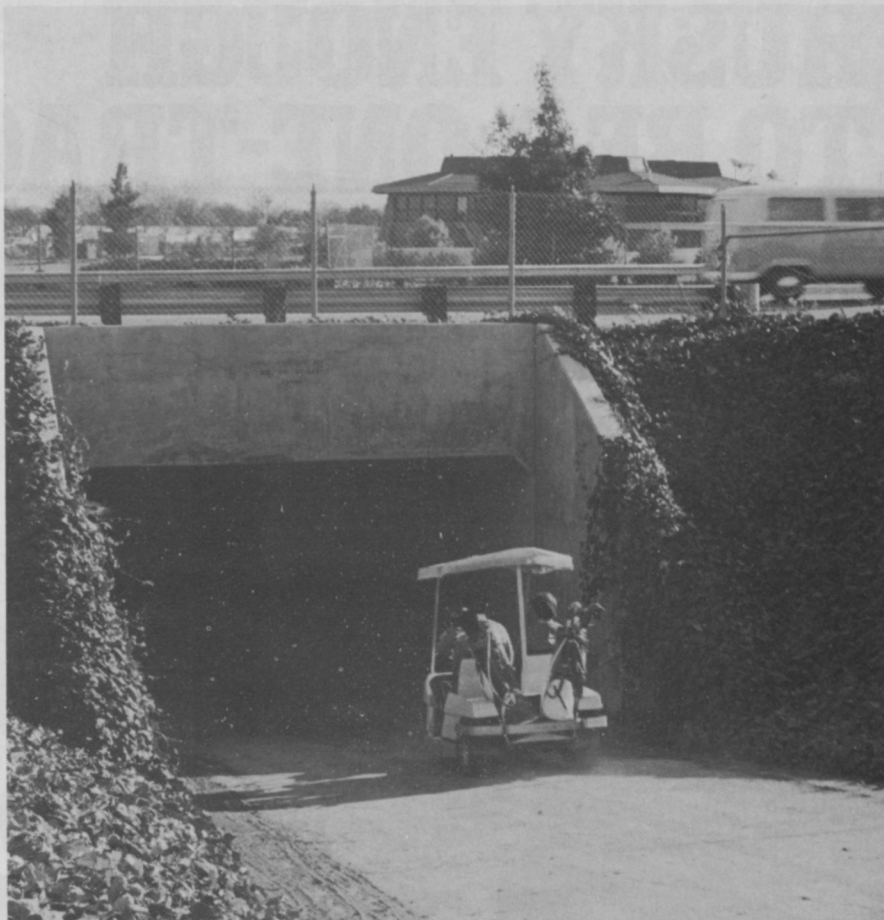
Safe from speeding automobiles above, golfers use the underground tunnel to connect holes 3 through 13 to the clubhouse side of the golf course.
