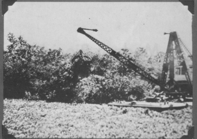
This photo taken on the north fork of the St. Lucie River shows a crane depositing hyacinths on the riverbank.
