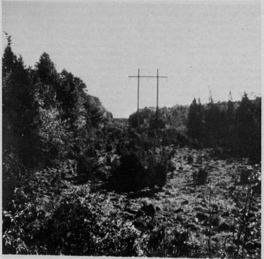
A 115 KV right-of-way under good control as the result of selective basal sprays. Ornamental steel poles are in background.
