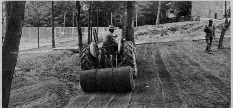
6. Rolls are easily transported and laid with a landscaping tractor.
