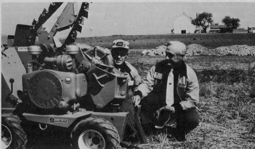
Edwin Malzahn, president of Charles Machine Works, Inc., right, discusses VP 12 unit with Warren (Doc) Jordan, president of Jordan-Kumler advertising agency at Oklahoma City. The 25 hp unit which lays both cable and irrigation lines has plow on front, and is built to fit the normal lawn gate.
