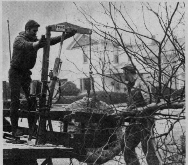
MOUNTED HYDRAULIC CRANE: Ruger Equipment, Inc., Uhrichsville, Ohio
