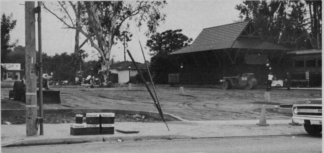
A typical parking lot is bladed to remove existing weed growth and compacted for better surface — prior to application of herbicide and asphalt. Pramitol 25E is applied on the \frac{1}{3} -acre parking lot below in less than an hour, with difficult areas sprayed by hand.
