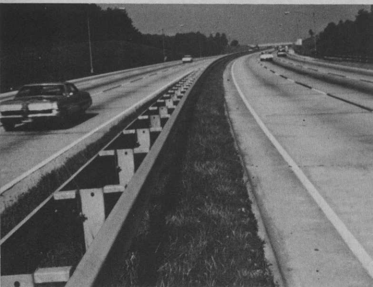
This median on a highway near Atlanta, Ga., was treated with 2 lbs./acre of MAINTAIN CF 125. In saving several mowings, it meant increased safety for workmen and traffic.
