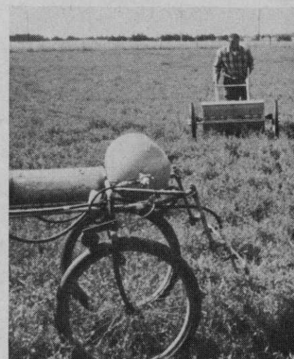
These are the spray rigs the Hancock Experimental Farm used in its herbicide trials on new forest plantings.
