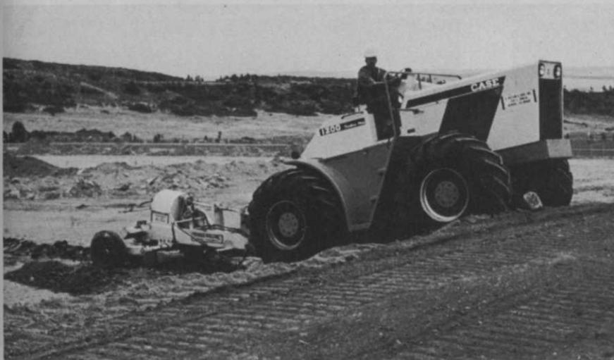
Kessen pipe-puller laying pipe. Puller works from a starter slit trench and pulls pipe through soil without trenching. On some jobs, puller can cut pipe placement time in half when compared to trenching.
