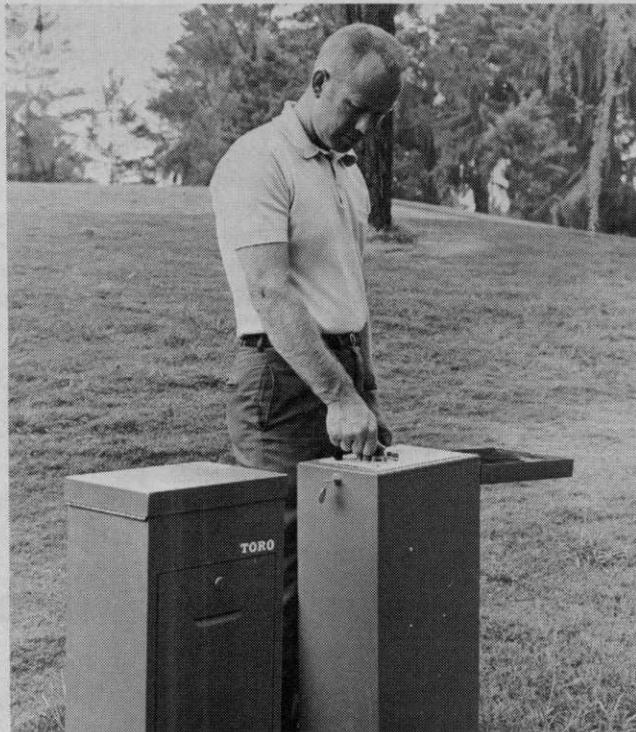
Greens Superintendent Arlin Grant manually adjusts a "satellite." The clock mechanism is connected to eleven sprinkler heads, and can activate each valve in sequence. Satellites are activated according to the program set at the central control panel.
