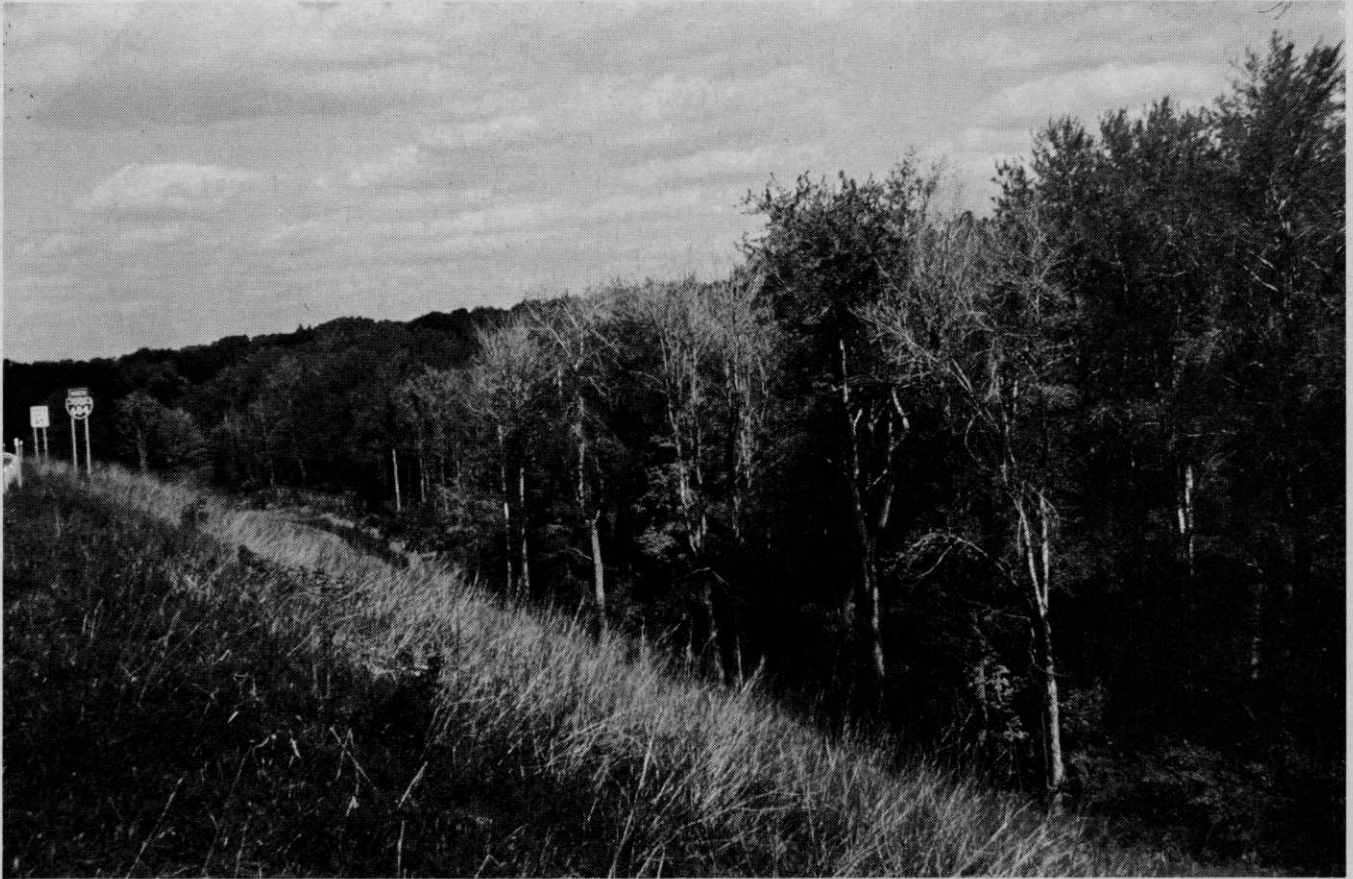
Trees nearest road are dying because of soil piled on top of root area during construction. These should have been removed.
