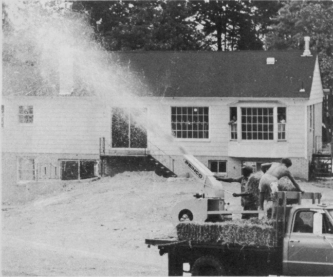
SKID-MOUNTED MULCHER, Reinco, Inc., Plainfield, N.J.
