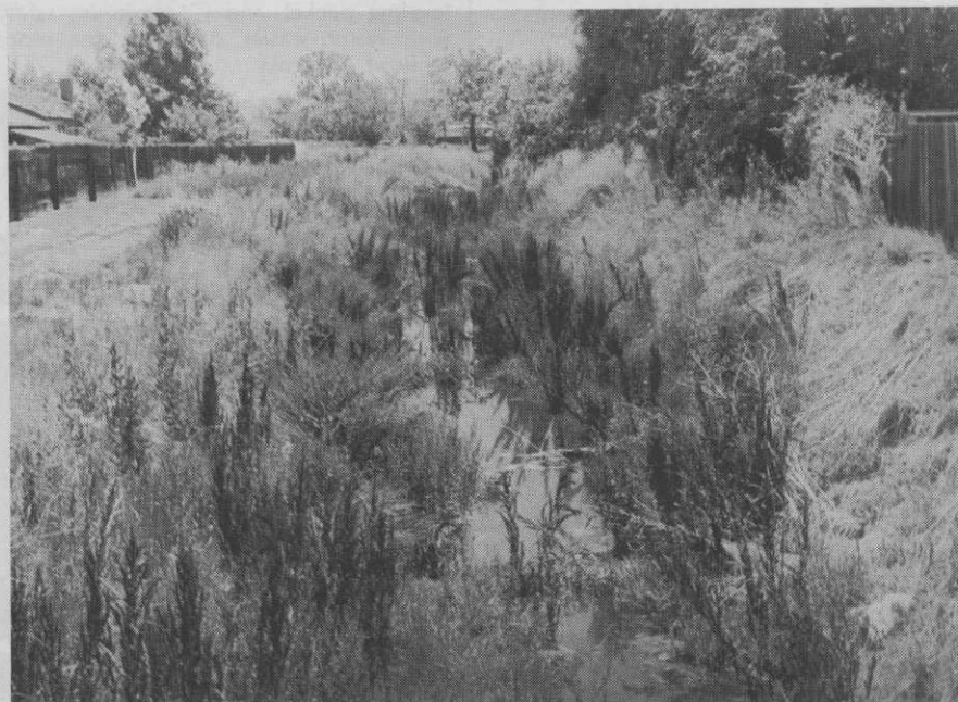
Weeds had harbored rodents, obstructed water flow, and created a fire hazard.
