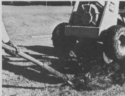
Pipe is attached to plow blade with cable pulling grip. The plow is then lowered into the hole and laying begins.
