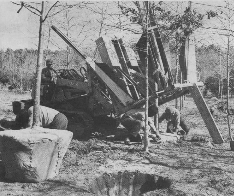
Big Vermeer tree spade cuts a clean package.
