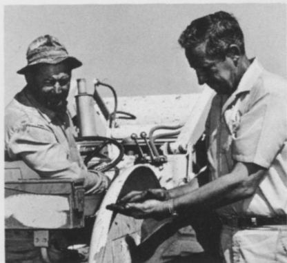
Harvey West, Jr. (right), developer of Graeagle, a vacation and retirement home community in Plumas County, California, discusses the sand-bark turf construction method with Carl Dell Aquila, contour grader.
