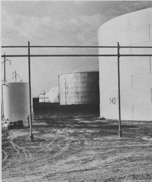
Bare ground around storage tanks from application of soil active herbicides eliminates fire hazard and boosts maintenance efficiency at petroleum refineries.
