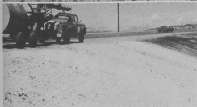
Pictured here is a plot mulched with green wood excelsior fiber at the rate of 2 tons/A. (Photo Four).
