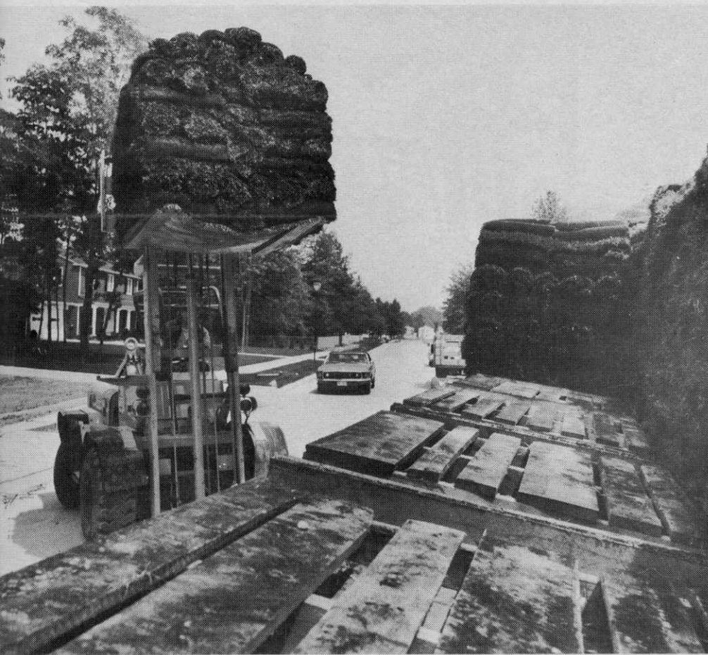
A full 100 yards of sod, supported by the wax-impregnated cardboard, is lifted from the truck and moved to the site in a simple one-man operation. The wood pallets stay on the truck.
