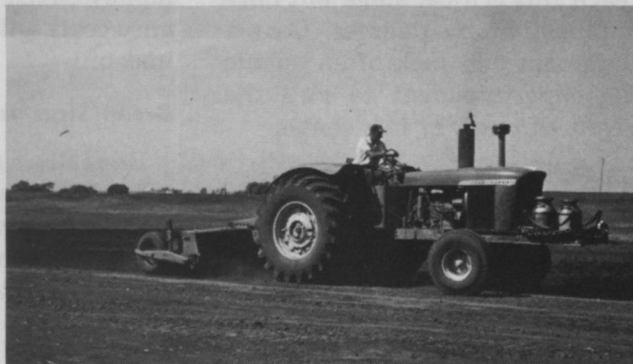
Step 4. Sand, peat, and topsoil are mixed thoroughly with roto-tiller. This final mix will be moved to green site and carefully spread to avoid compaction.
