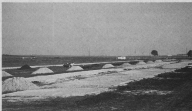
Step 3. Calculated amount of sand was dumped beside mixing strip prior to spreading. Then sand (1½ inch depth) was placed on top of peat. Doing work in strips facilitates mixing with equipment.
