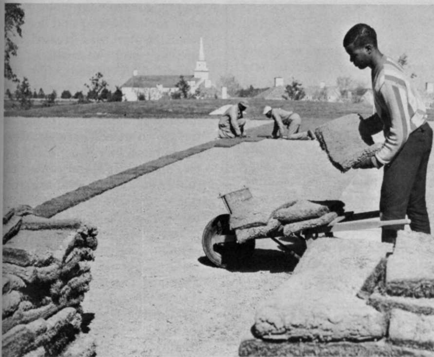
Rossmoor Leisure World's sod is carefully installed on this section of the 120-acre golf course. As summer drought cancelled hopes of the grass seeding on its own, 79 acres of turf was ordered to carpet fairways and greens. Only grass in the roughs will be left to rely on nature.
