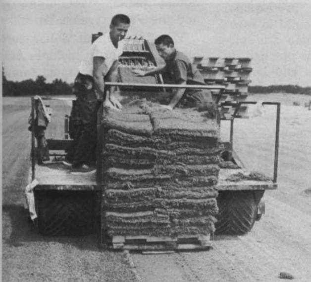
Loaded pallet from sod harvester is lowered and automatically slides into position on field to be picked up by forklift and loaded for transport. Employees are, left, Fran Hurley, and Oleboreo Miranda.
