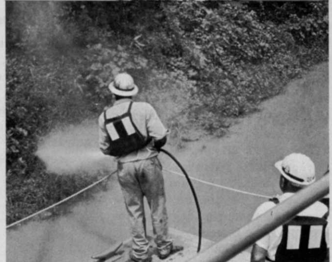
Barge from which 500-gal. batches of chemical-water mixture are sprayed can cover 6 miles a day.
